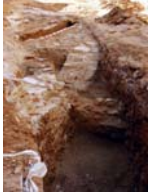
PIC00929 Vista general sector excavat
