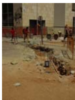
PIC01839 Vista general sector
