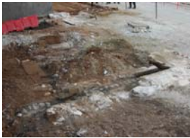
PIC02083 Vista general final
